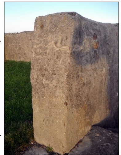
The benchmark can be seen near the base of the front of this end-of-wall
